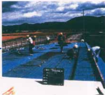
2. Slab is placed on EPS block and concrete is cast.
