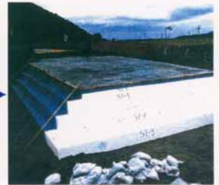
3. Fill is completed upon execution of sub-base course work.
