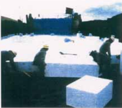
1. Stacking of EPS Blocks
